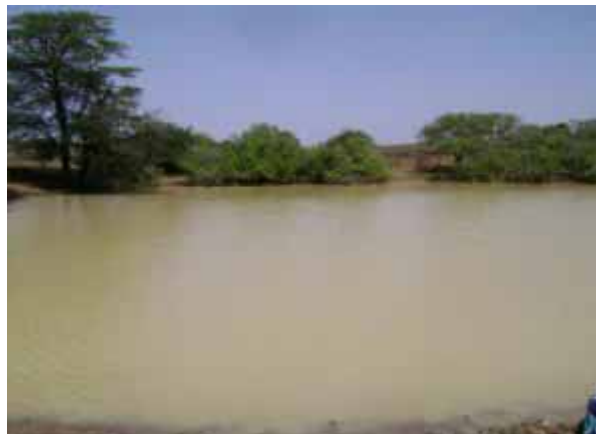
Fully replenished Asha-Gabo communal dam – Baidoa- Bay Dec. '09
