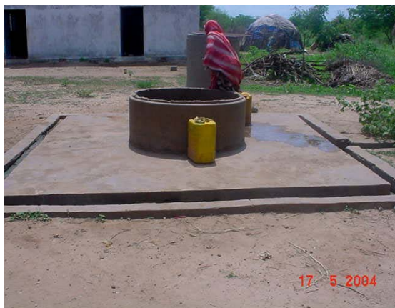
Makayuni and Gumayni wayney villages hand dug wells. AFREC has rehabilitated them and are ready for hand pump installation
