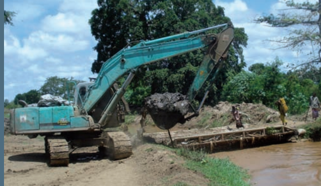
Mechanised rehabilitation of a primary canal in Merka. Photo: FAO Somalia
