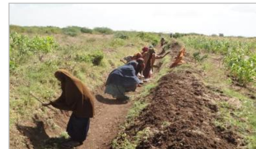
Canal Rehabilitation for the Coming Season. Qoryoley, Lower Shabelle, FSNAU, Dec. '10
